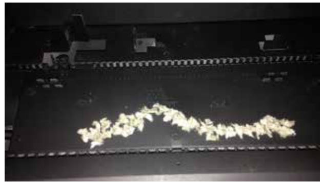
Figure 12 - Installing the glowing embers (BV32 Shown)
