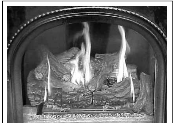
Figure 30 - Burner Flame Appearance
