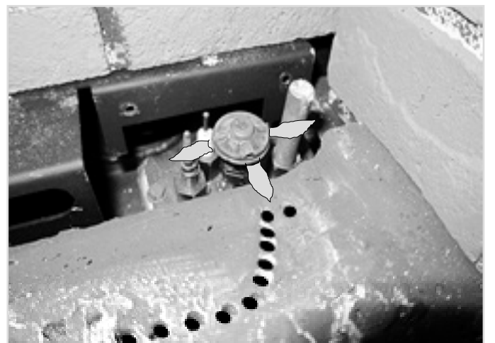
Figure 48. Use caution in placing the logs to ensure that the pilot carry-over ports are not obstructed.
